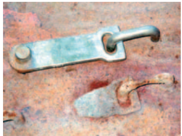
The photo shows an original 25:20 steel component and the same component coated with 53-606 after 12 months in service.
