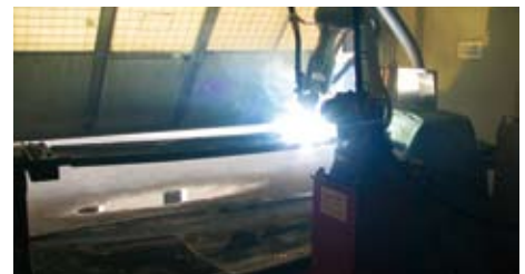
Coating with Automated Unit
